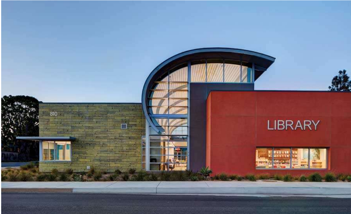
A large, central, wave-shaped roof runs the length of the 14,830-sq-ft Imperial Beach Library. Photo by Stephen Whalen
